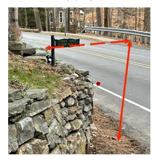
Exhibit 30: View of Route 148 reverse curve looking on Route 148 westbound. Note the limited visibility around the curve, and the limited shoulder width on the northern side of the roadway. (Source: Google Maps)
