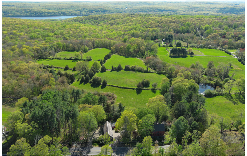
Drone image showing the Palmer-Warner House (bottom right), the fields, and the Connecticut River.
